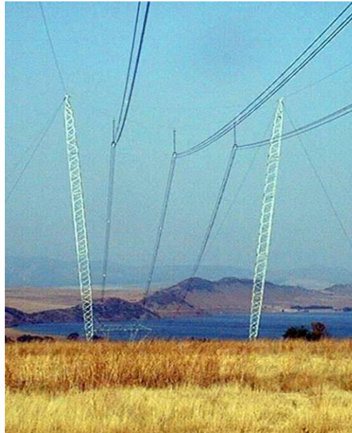
Figure 48.11: Crossrope Suspension for TX lines
