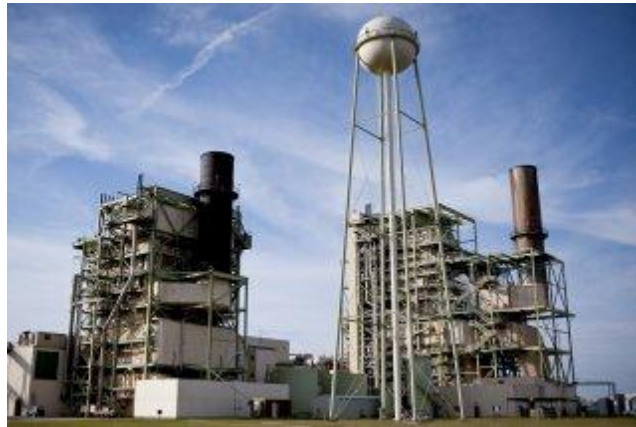
Figure 38.6: 100-MW gas-fuelled power generation plant
