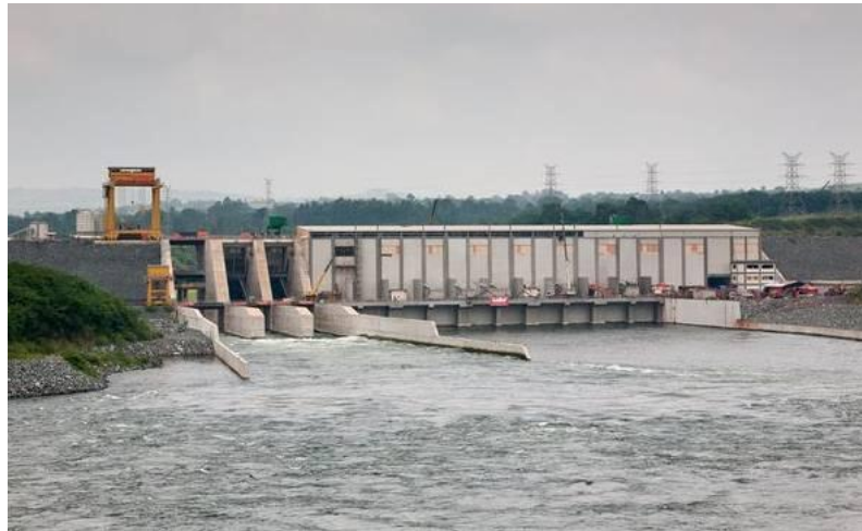
Figure 53.2: Bujagali Falls project
