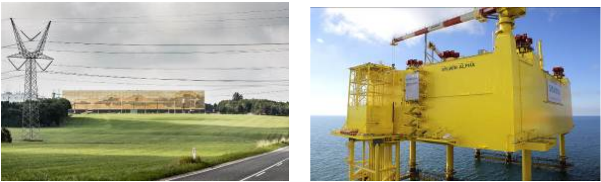
Figure 1. a) The 700 MW, 500 kV Skagerrak VSC-HVDC converter station connecting Danish wind with Norwegian Hydropower. [Copyright ABB] b) The 864 MW off-shore VSC-HVDC platform Sylwin Alpha after installation [Copyright TenneT]
